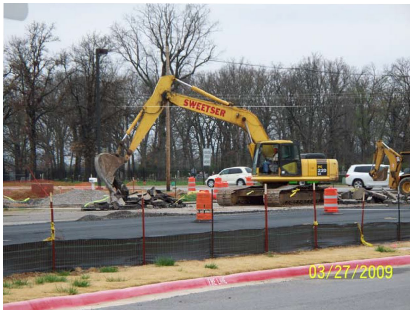
Photograph CS-4 – Example of Silt Fencing
