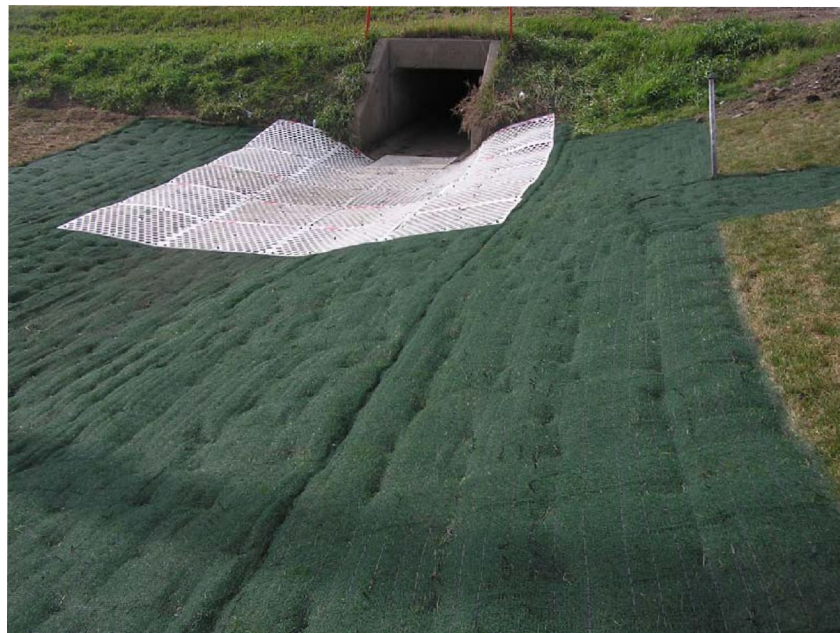
Figure CB-10 – Typical Turf Reinforcement Mat Application (Scourstop.com)
