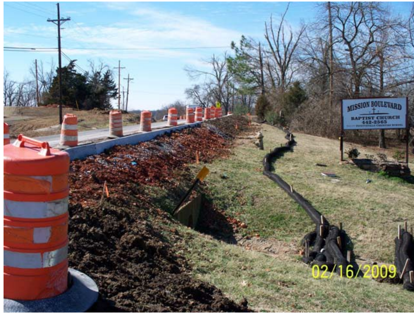
Photograph CS-7 – Example of Fiber Roll/Wattle
