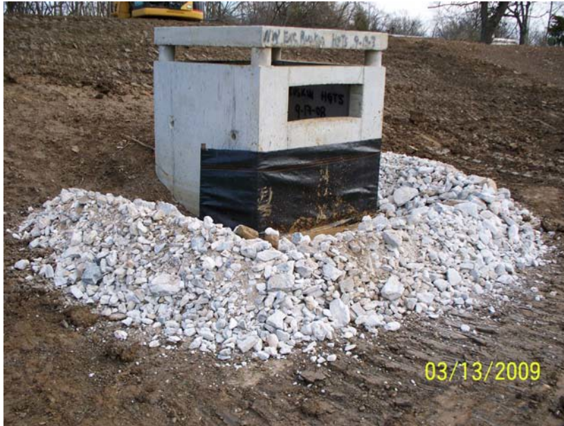
Photograph CS-5 – Example of Inlet Protection
