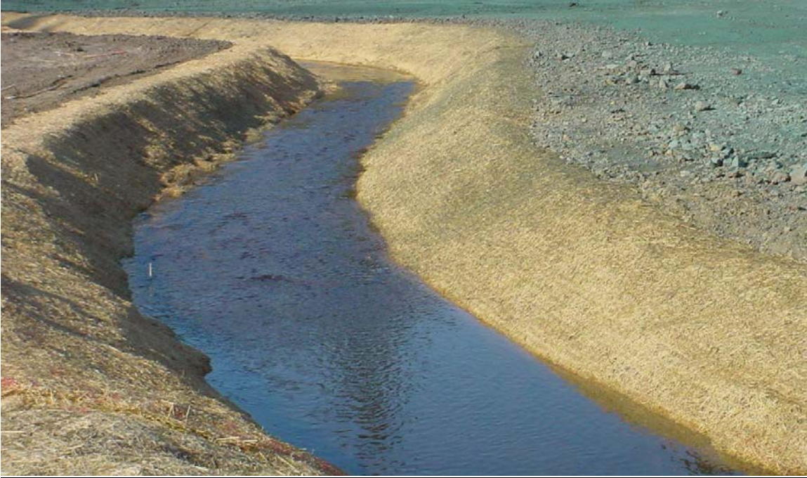
Photograph CS-3 – Example of Erosion Control Blanket
