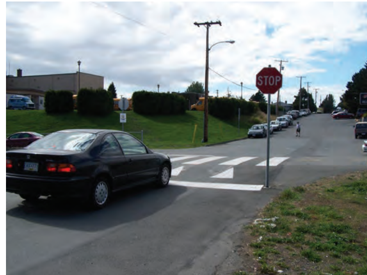
Raised crosswalk at an unsignalized intersection.
