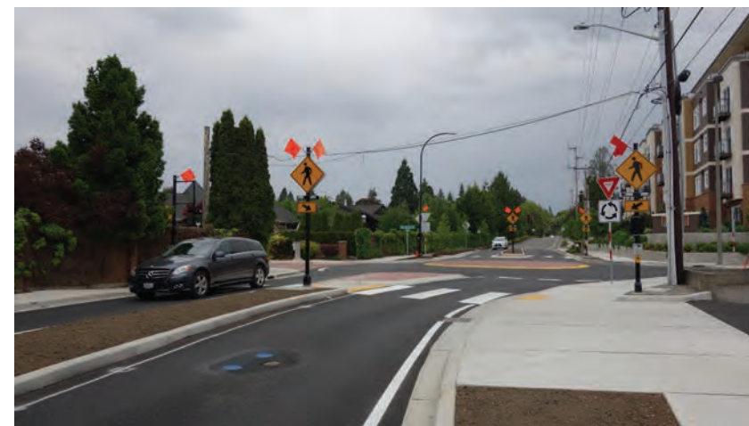
Roundabout approach with median and splitter island, and street crossing
