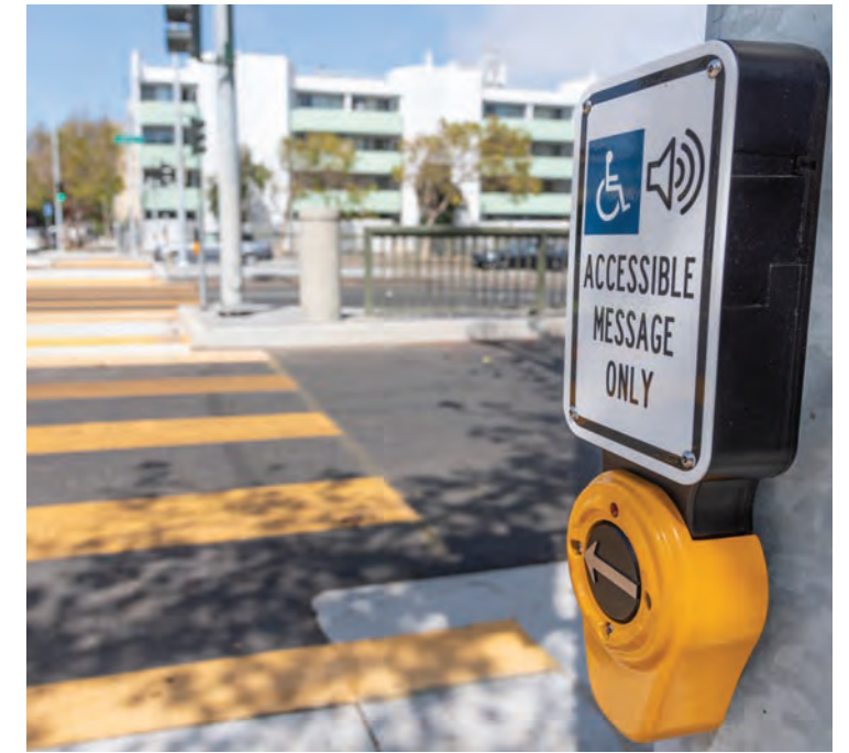
Accessible street crossings at a signalized intersection
