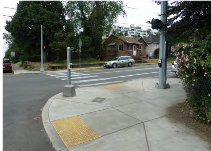
Curb ramps and pedestrian signals provide safe, accessible routes for each crossing direction
