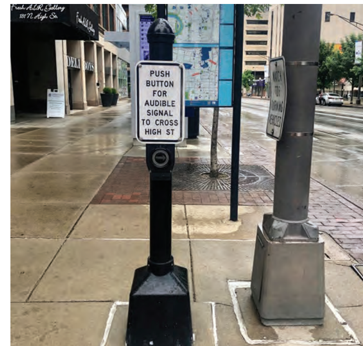
Accessible pedestrian signal button and signage
