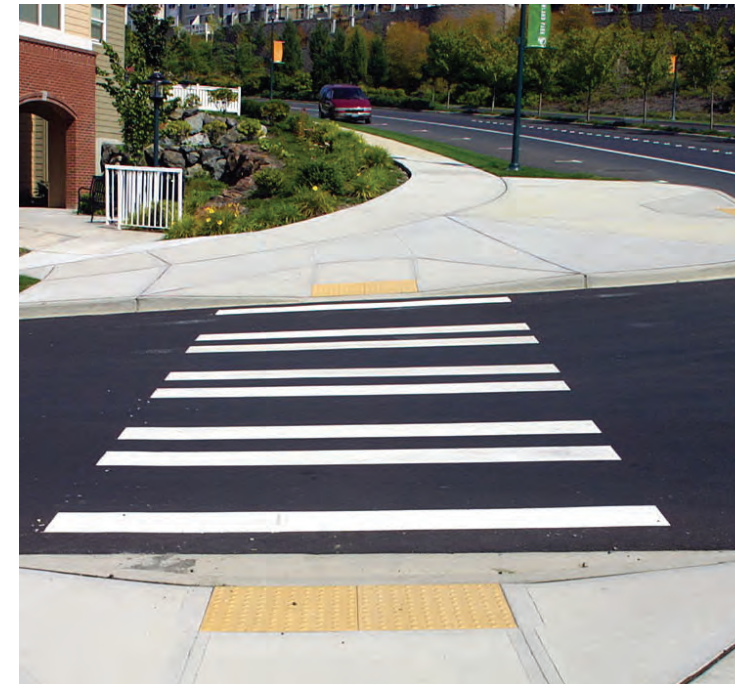
Accessible street crossing at an unsignalized intersection
