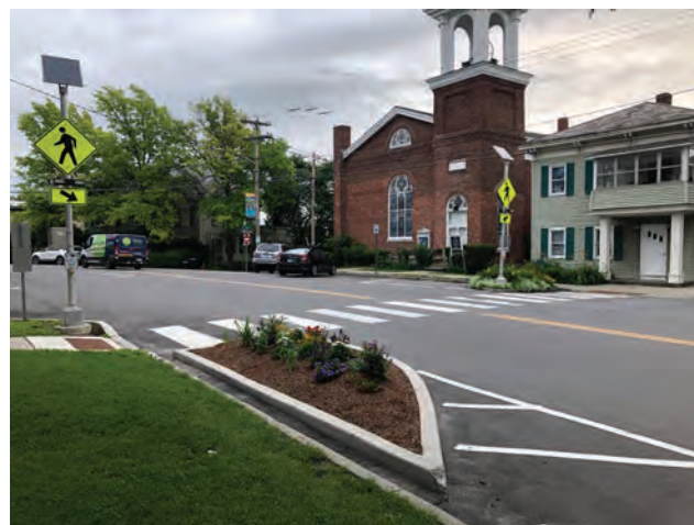
Visual narrowing using landscaped curb bulb outs. Channel is maintained for drainage.
